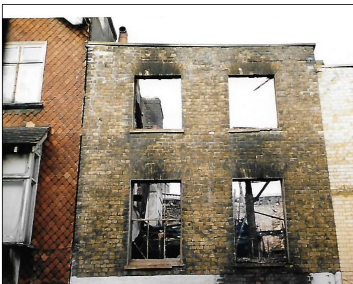
Showing the extent of the fire damage to 52 High Street in 1992. The High Street was closed for six months whilst the rebuilding work took place
